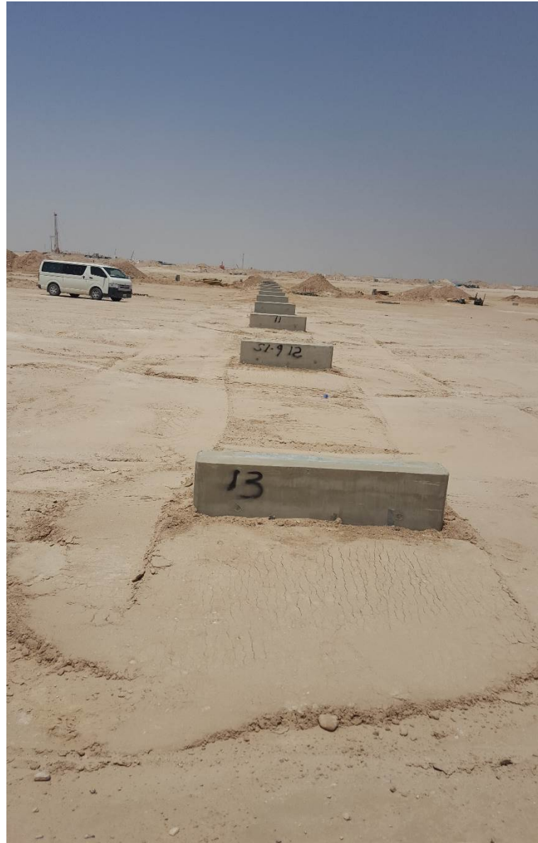
KOC - LFHO - Pipe Sleeper Installation
