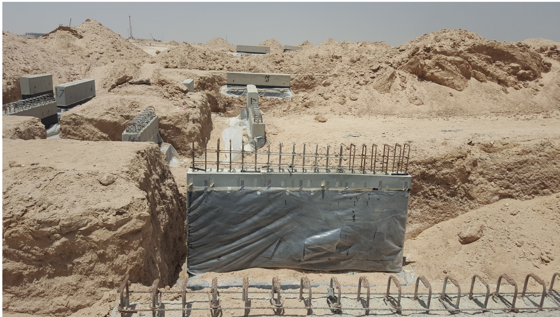
KOC - LFHO - Pipe Sleeper Installation
